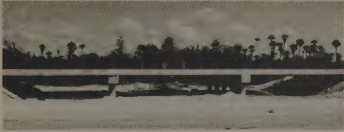
From Naples to Fort Lauderdale, State Road 87 is known as Alligator Alley. Its replacement by Interstate 75 includes thirty-six underpasses like this one, strategically placed to permit water flow and provide safer crossings for wildlife.
